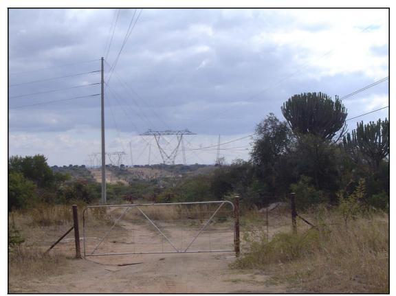
**Figure 10:** Existing Matimba-Witkop 400kV transmission lines (Note: The vegetation cover is removed underneath the power lines).
